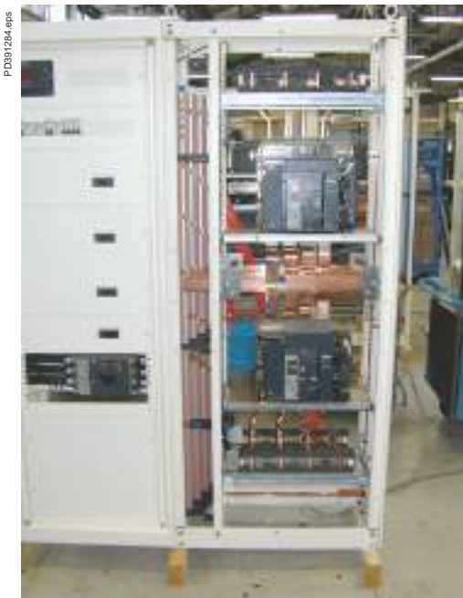
Source changeover system in 2 combined cubicles.
