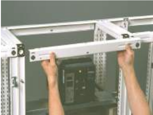
Cross-pieces can be removed to facilitate work.
